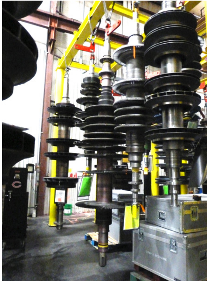
Climate-controlled rotor storage facility ensures spare rotors are immediately available.
