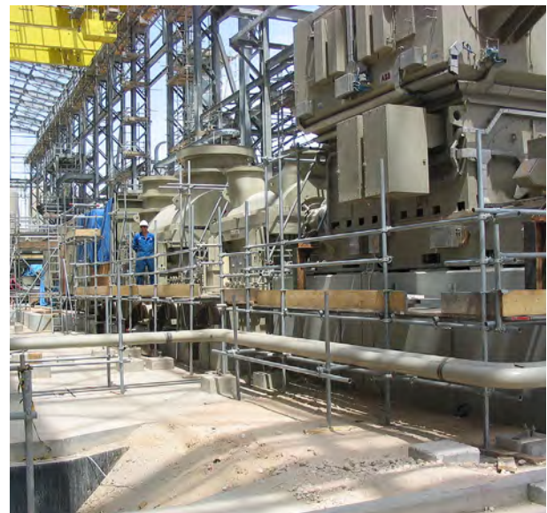
88M4 & 60M4 mixed refrigerant compressors.
