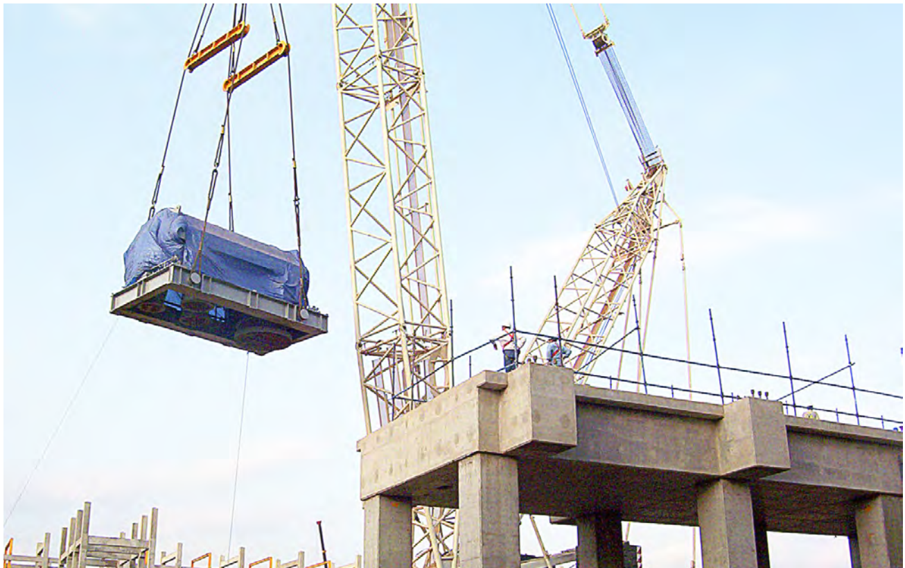
88M6I LP/MP mixed refrigerant compressor.
