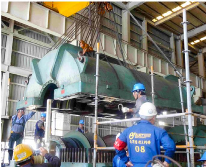
An Elliott field service crew removing an upper compressor casing.
