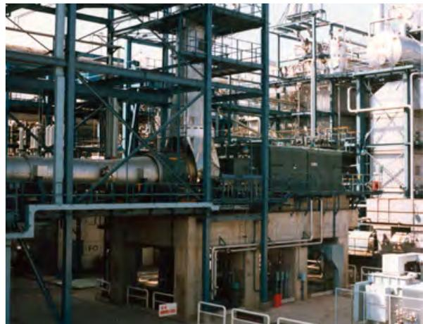
Site installation of an expander power recovery unit.
