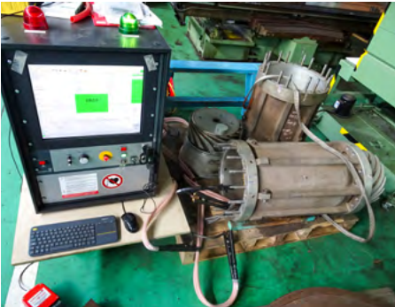
Stator electrical test.
