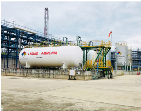
Liquid ammonia storage used in food production.
