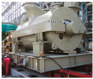
**Figure 6.** Installation of a large propane compressor with three side streams in the Middle East.
