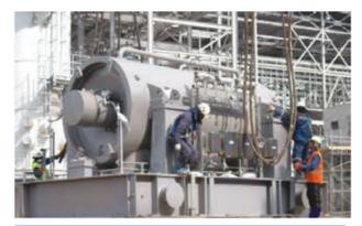
**Figure 1.** Installation of an Elliot 60MB61 LNG mixed refrigerant compressor in Russia.
